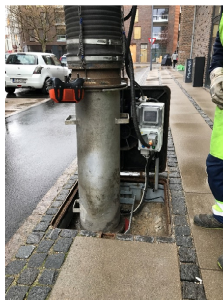
Figure 35 - Emptying via a flush recessed suction port
