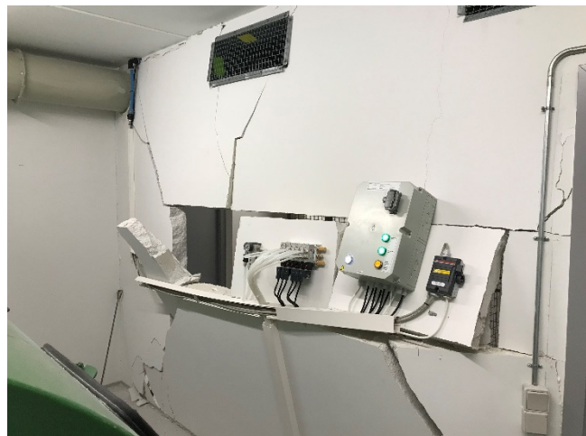
Figure 28 - Wall cracked due to lack of replacement air.
