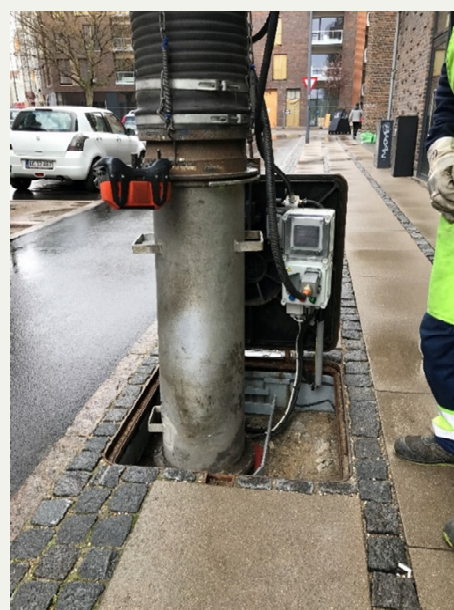
Figure 35 - Emptying via a flush recessed suction port
